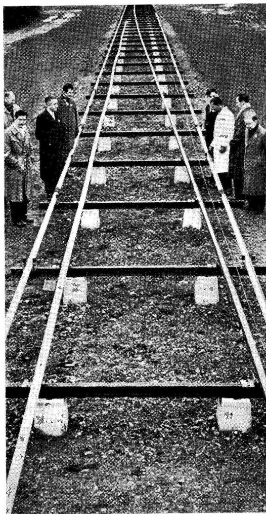
On January 31, the Institution of Electrical Engineers held a convention on Long-Distance Transmission by Waveguide, a method by which a very wide band of frequencies can be accommodated. In the system developed by Standard Telephones & Cables Ltd. at their Enfield laboratories, the waveguide is a hollow copper tube of circular cross-section, which must be laid optically straight. Using P.C.M. (Pulse Code Modulation) the actual capacity of the waveguide system, as shown here for demonstration at the convention, is some 400 separate television channels. This marks a very considerable advance in wide-band transmission systems and makes a Trans-Atlantic TV pipe a feasible proposition.
